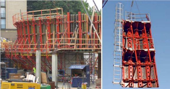
Figure 8: PERI RUNDFLEX formwork prepared for a lift pour Figure
