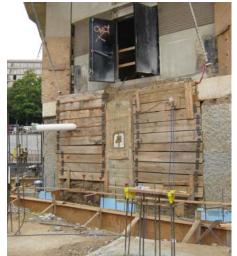
Figure 13: Underpinning - interpier beam/wale system (Fichandler)
