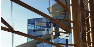
Figure 10: Parallel Strand Lumber Columns with support arms and muntins
